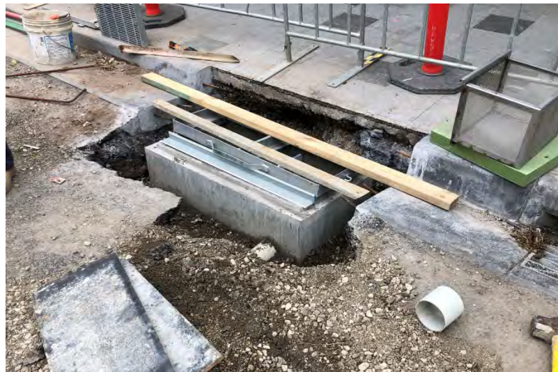
SVC Catch Pit for sediment and litter capture prior to infiltration systems
